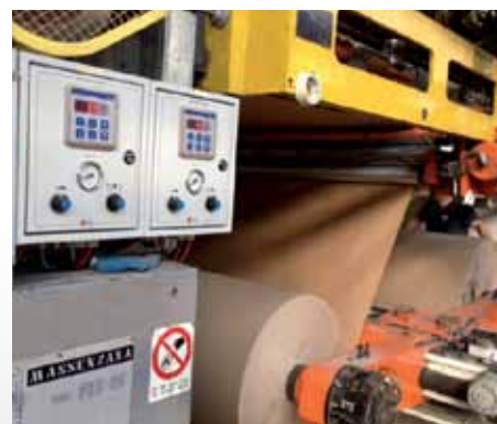
ReTens su corrugatore ReTens on corrugating plant
